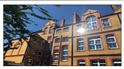
Every Project Counts were contracted by the London Borough of Newham to carry out the extensive repairs and restoration of the exterior of Ranelagh School including new double glazed windows, stonework, tuck pointing and gutter repairs.
