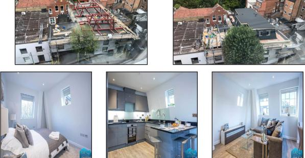
The Scheme involved building a steel frame structure on the top of occupied flats below in a central London location. This presented our site team with many challenges which involved road closures for lifting equipment, temporarily re housing of occupants and liaising with adjoining owners regarding Party wall matters.
